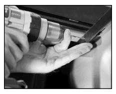
G. Adjust header bar as directed in Step 1D and fully tighten bolts. When header bar installation is complete, proceed to Step 3 of special toolbox instructions.
