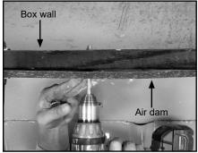
D. Insert carriage bolt through air dam and box wall.
