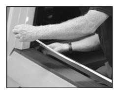
C. With side rail set on top of box, position side rail tight to front of box. Working from front of box to rear, adhere side rail to inside edge of box rail.
